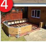
Attach brick skirt and modular wall to steel base and finish by fixing the bridging tiles in place.
